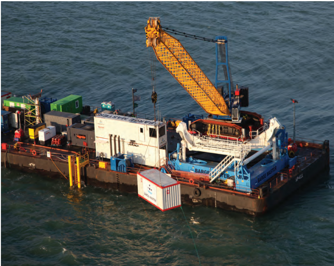
Barge Master T700 supporting crane operations in the North Sea
