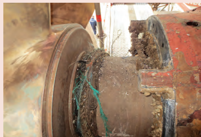
Typical netting and rope around rotating shaft damages aft seal.
