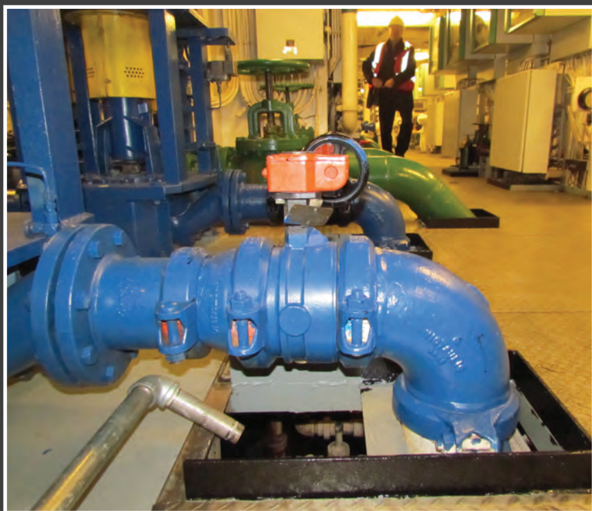
Couplings are most effective in attenuating noise and vibration.
