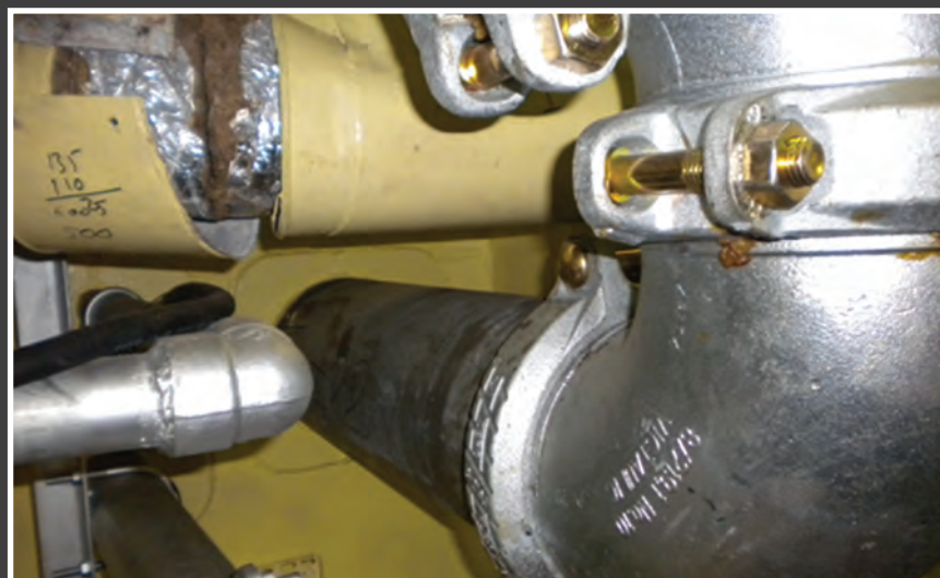
Weight reductions by using grooved pipe couplings instead of flanges are achievable across a range of pipe sizes.
