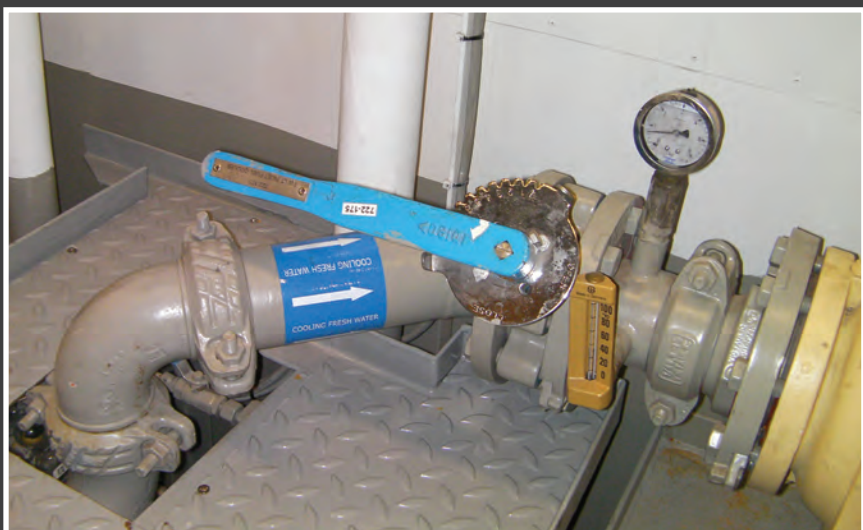
Deck penetration: the small size of grooved components makes them ideal for jobs where space is limited.
