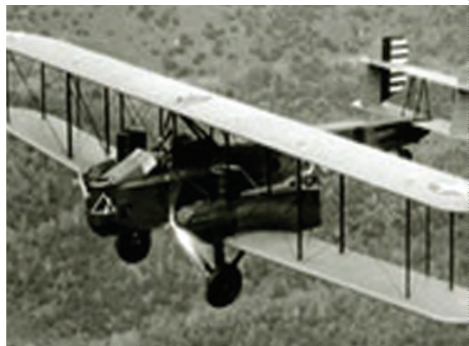
Below: Predecessor of the modern Drones? Pilotless plane controlled by Sperry gyroscopes, a pilotless Curtiss B-2 flies over Sacramento, Calif., in May 1930.
