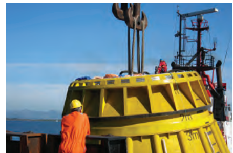
Lifting of FPSO loading turret.
