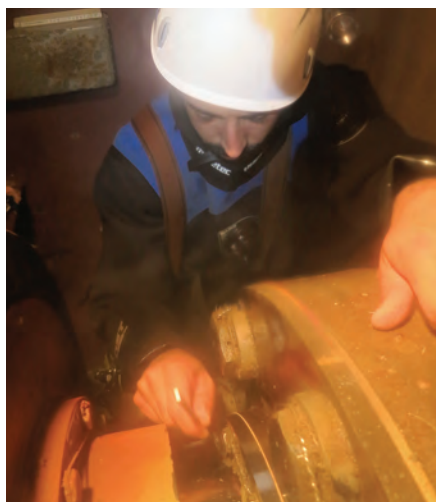
Diver/technician working on the shaft seal assembly.
