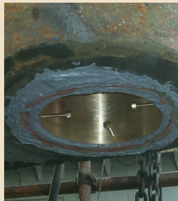
Picture 5: Finished application after injection of Belzona 1321
