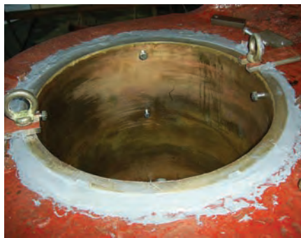
Picture 2: Bearing housing installed using composite materials
