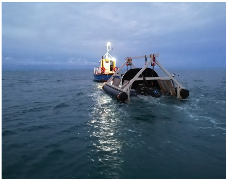
Installation of the prototype near Hanstholm.
