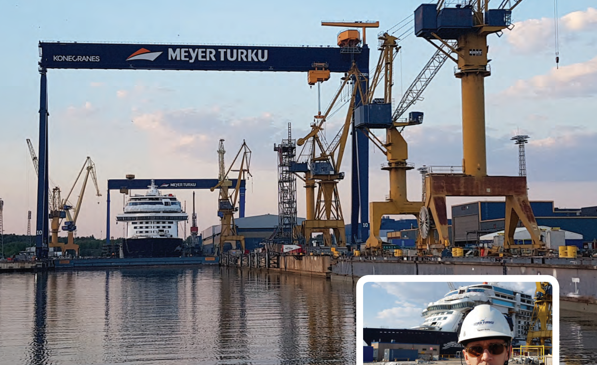
Above: Meyer Turku Shipyard, one of the world's largest builders of cruise ships. The new huge 1,200t gantry crane is about to be taken into use. The outfitting now takes place in all areas on-board. The yard area covers 144 hectares and the dry dock measures 365m x 80m.
