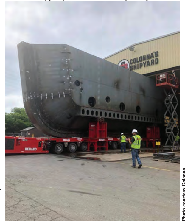
Colonna Shipyard/Caisson for USN graving Dock
