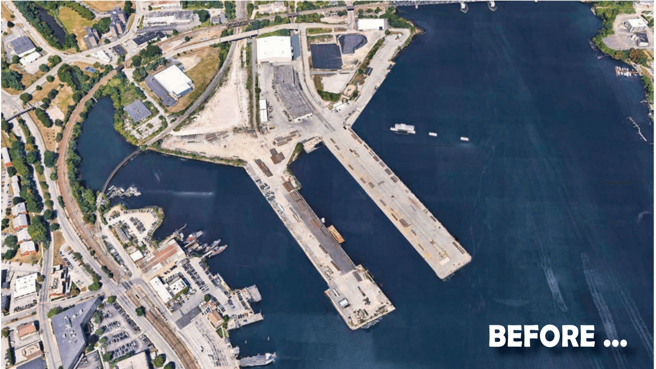
Images Courtesy of Connecticut Port Authority. Rendering Artist: Jennifer Gottlieb, AIA NCARB ENV SP at AECOM
