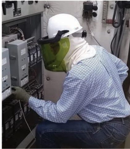
Figure 7: One of the Authors with Arc Flash PPE Protecting up to 12 cal/cm² (including special arc flash gloves, shirt and jeans)
