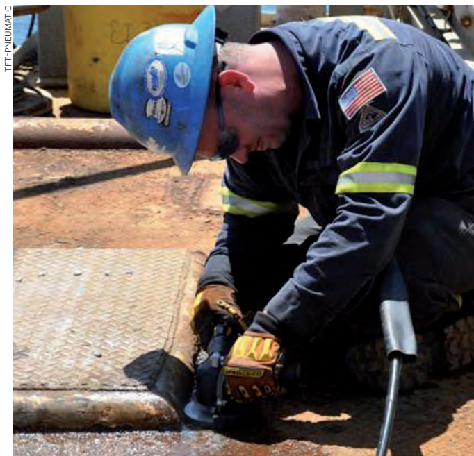
Spark-less cutting tools are available to eliminate fires from hot work.
