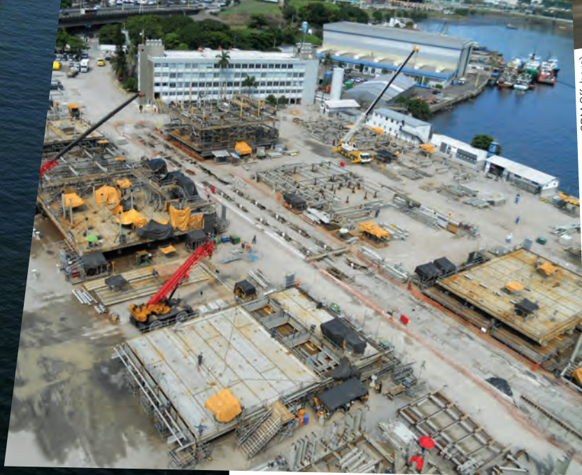
Overview of modules under construction at the Brasa yard in Niteroi.
