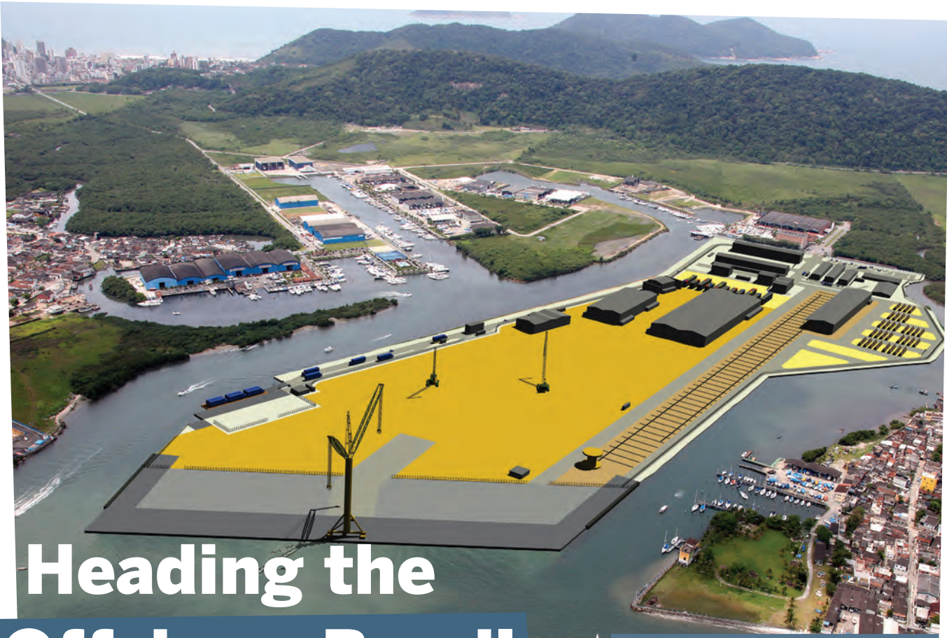
Aerial photo of the new fabrication site
