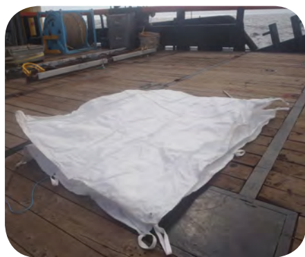
Fabric bags are filled with grout as seabed supports.
