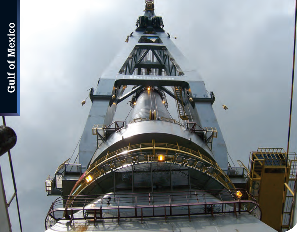
Subsea 7's construction vessel Seven Borealis had its 5,000mt offshore mast crane installed by Huisman in Schiedam, Holland, in 2011. (Photo: Huisman)
