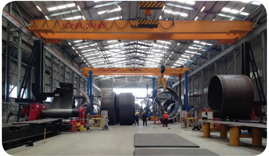
TAG Energy's production hall on Teeside creates offshore wind farm monopile and transition pieces with a 24/7 operational linear manufacturing line.
