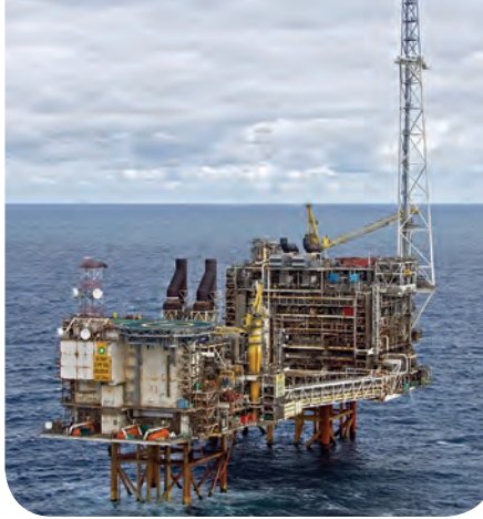
Eastern Trough Area Project central processing facility.
