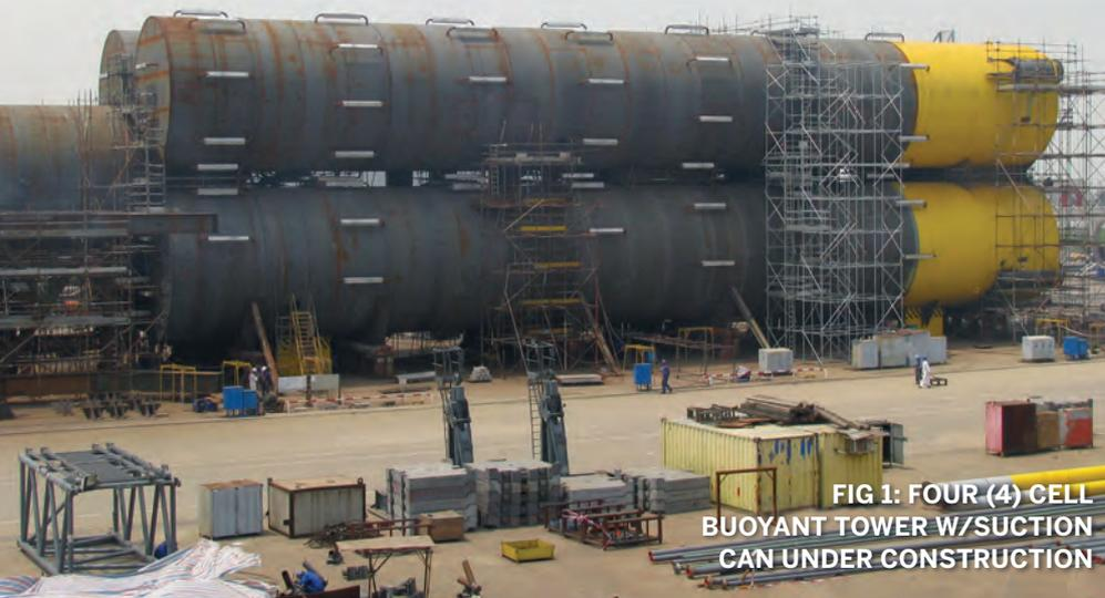
**FIG 1: FOUR (4) CELL BUOYANT TOWER W/SUCTION CAN UNDER CONSTRUCTION**
