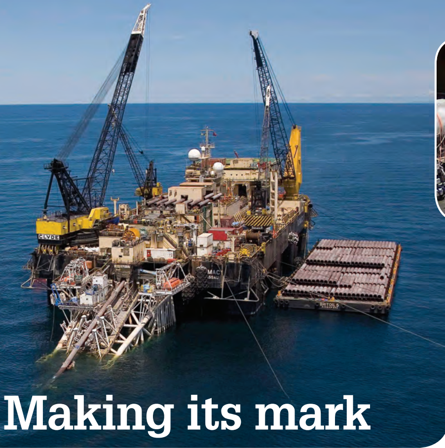
Above, the offshore and onshore pipelines are tied-in at the Omati landfall. Saipem's Semac 1 , left, is shown during deepwater installation.
