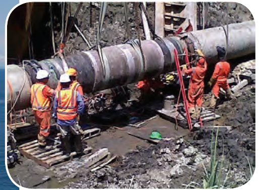
Above, the offshore and onshore pipelines are tied-in at the Omati landfall. Saipem's Semac 1 , left, is shown during deepwater installation.
