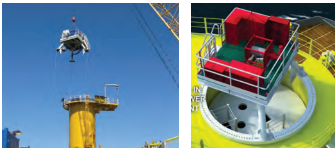
Left — Technip’s pull-in module, being lifted onto a transition piece on the Lincs Wind Farm, offshore Lincolnshire. Right — A visualization of Technip’s pull-in module. Images courtesy of Technip.
