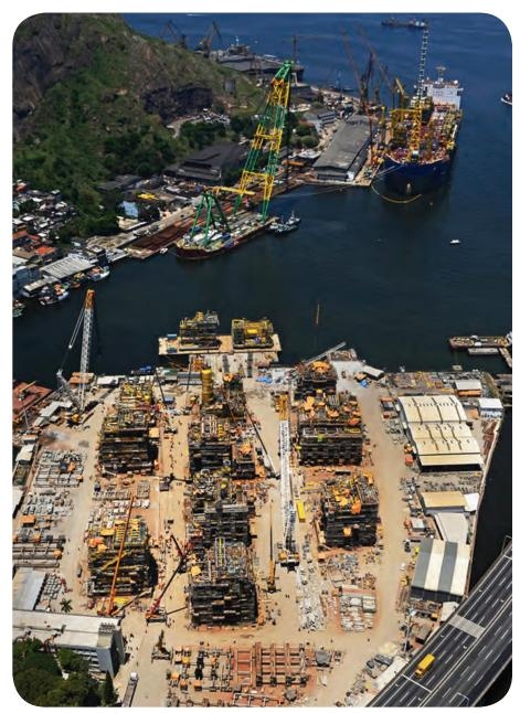
and injections modules, along with all the redundant safety systems required for such a vessel. Once the module integration is completed the vessel will be installed on the Sapinhoá presalt field, spread moored at a water depth of 2140m.
