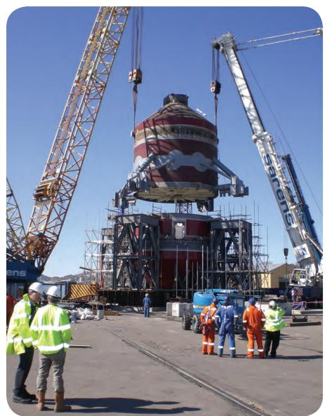
Ocean Resource's production buoy concept under construction. Photo from Ocean Resource.
