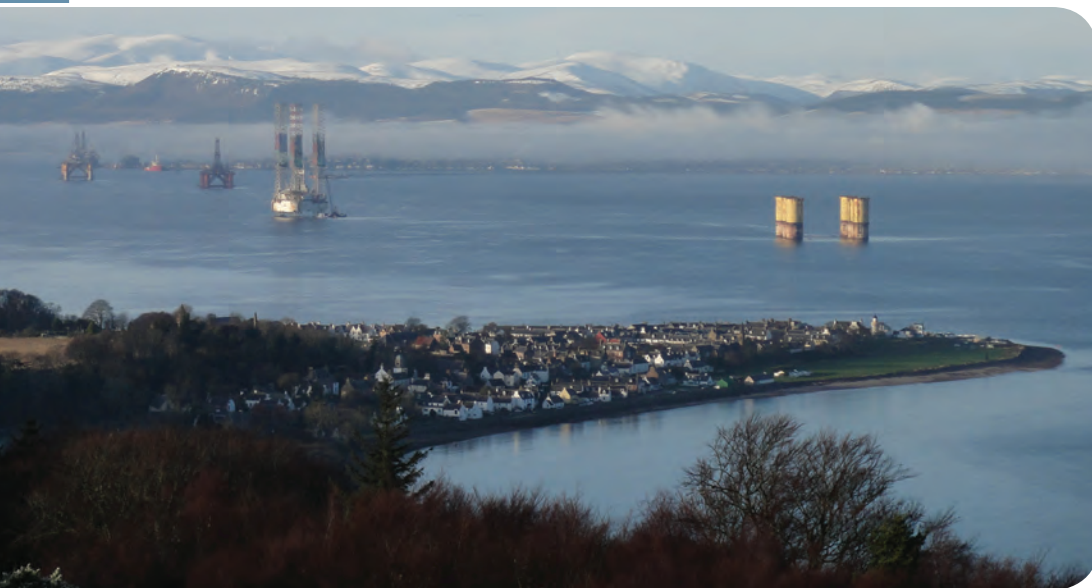
Hutton TLP legs—the first TLP installed—at Scotland's Cromarty Firth, post field decommissioning.
