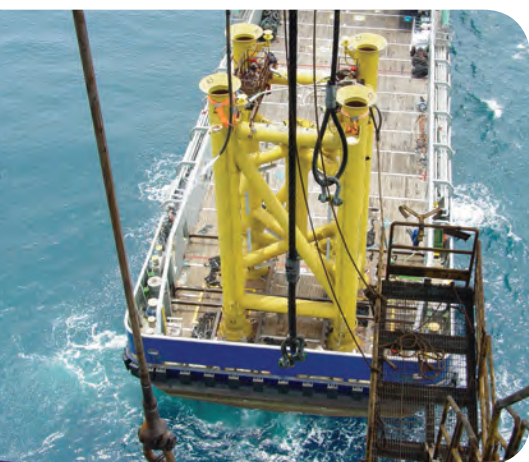
Subsea structure ready for installation using the Noble Tommy Craighead jackup drilling rig.
