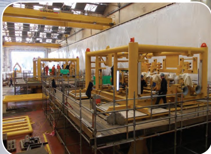
Two SSIVs in a fabrication bay.
