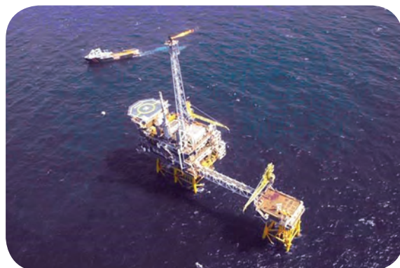
Offshore Energy Tier II Compression Project, Offshore Nova Scotia. Photo from SNC-Lavalin
