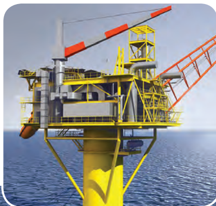
Articulated tower concept. Images from Atkins.
