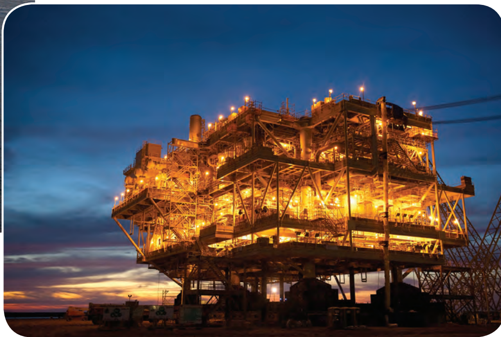
The deck of the Tamar platform, shown in 2012, while under construction.
