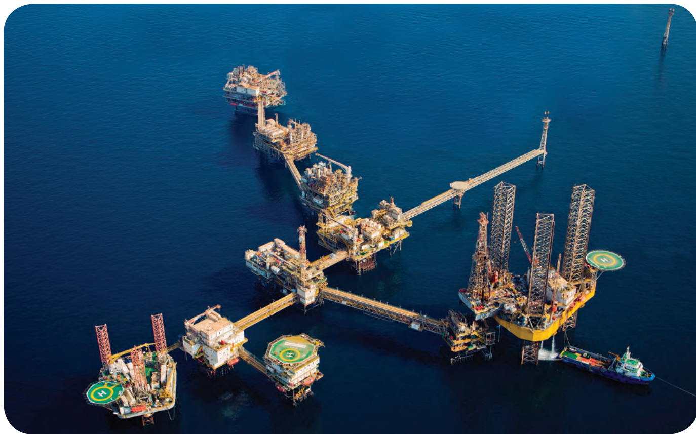
The Abu Al Bukhoosh central facility, operated by Total, offshore Abu Dhabi. Photo from Total.
