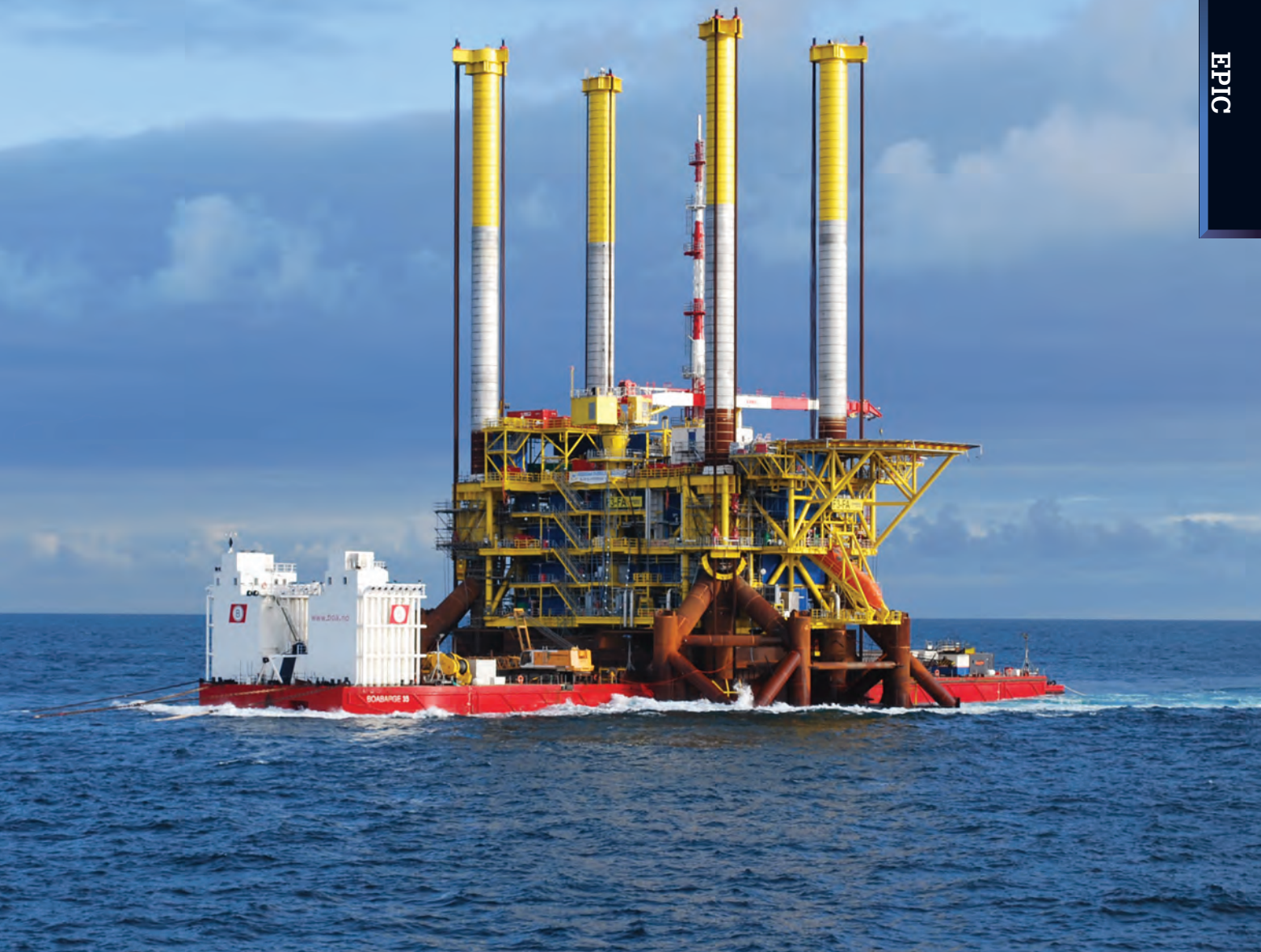
Centrica's F3-FA self installing platform being transported offshore. Image from Orca Offshore.
