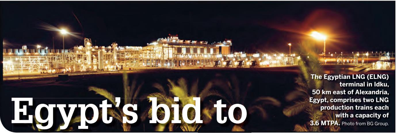
The Egyptian LNG (ELNG) terminal in Idku, 50 km east of Alexandria, Egypt, comprises two LNG production trains each with a capacity of 3.6 MTPA. Photo from BG Group.
