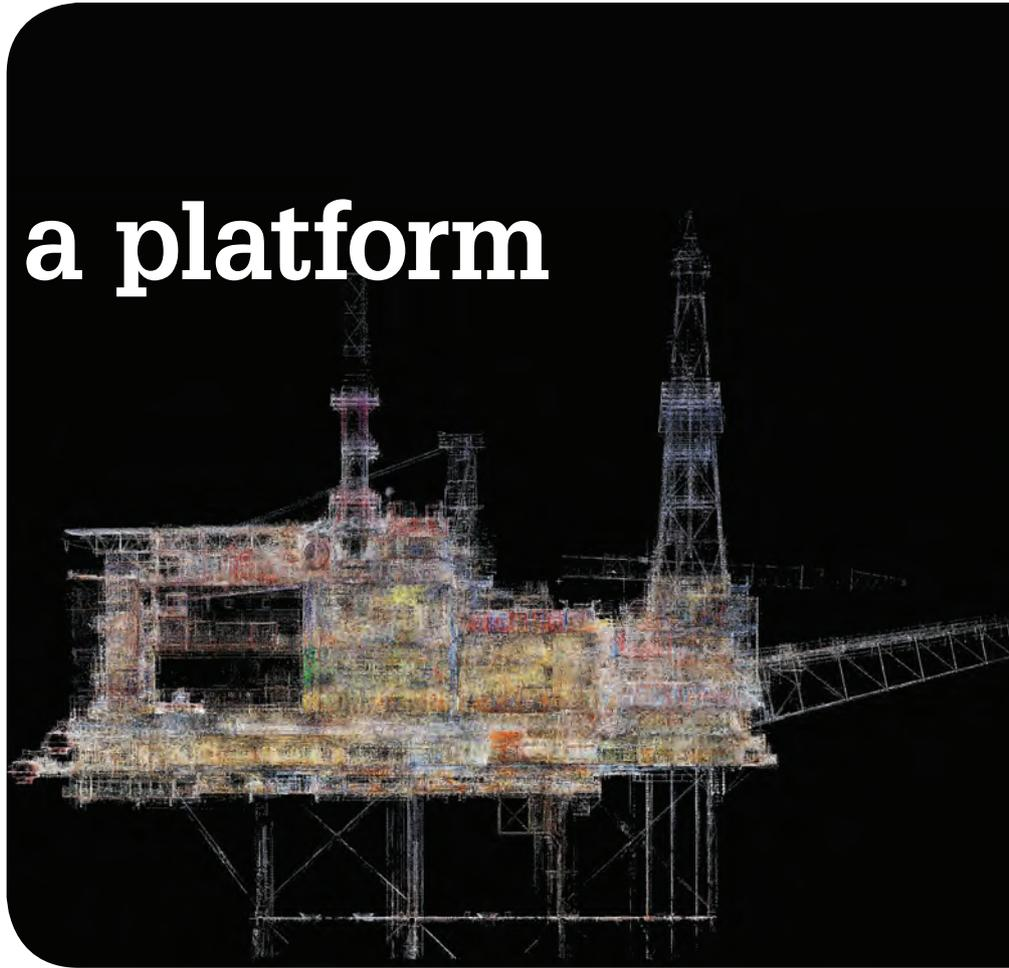
accuracy is degraded above that distance. However, during processing, the ODL dimensional control survey (DCS) team filters out all scan data beyond 15m, improving the accuracy, reducing the amount of data to be processed, and removing returns from distant spools or modules that would show up as noise.
