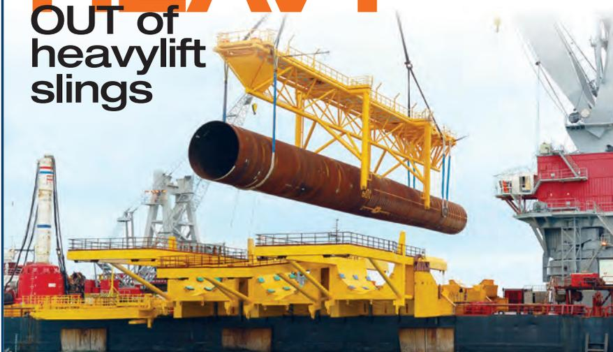
*Greater Gabbard Project: The world's largest wind farm. Seaway Heavy Lifting installs turbine monopiles with Samson's AmSteel<sup>®</sup>Blue lifting slings.*
