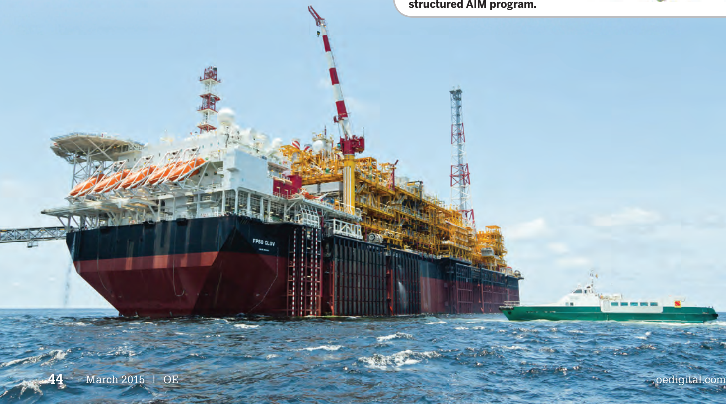
CLOV Hull and Topsides integrated model in as-built state as a foundation for a structured AIM program.
