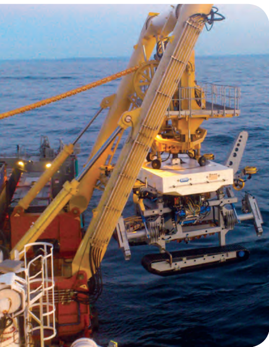
Launching the Fugro Q1400 trenching system. Photos from Fugro Subsea.
