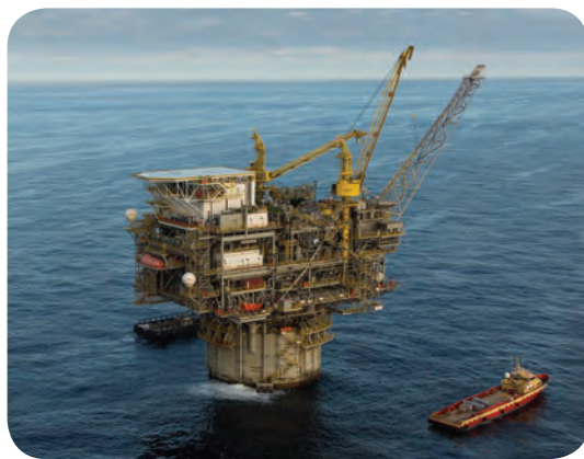
Anadarko's Lucius Truss Spar, located in 7100ft of water, in Keathley Canyon 875, 236mi offshore in the Gulf of Mexico. Image from Anadarko/Robert Seale.
