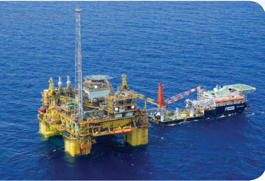
Gumusut Kakap, which came on stream in October 2014, was Shell's first deepwater project in Malaysia in 1200m water depth. Photo from Shell.
