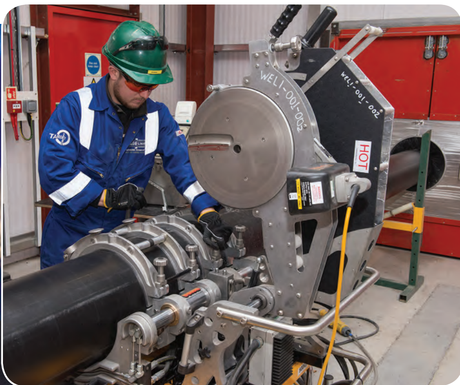
Butt fusion welding of polymer pipe. Photos from Swagelining.
