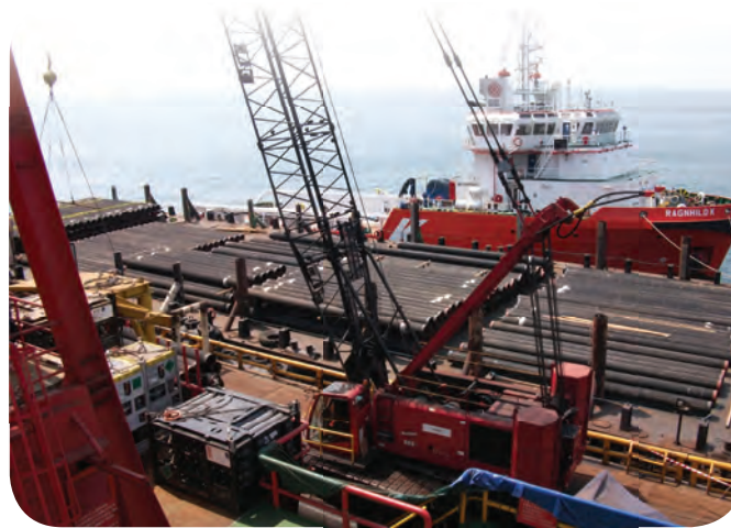
Pipes being unloaded from a supply barge to the pipelaying vessel.
