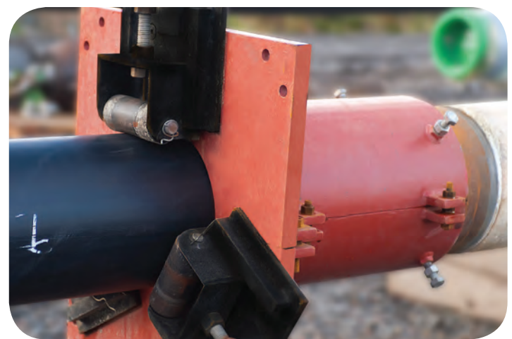
installation of polymer liner into steel string.
