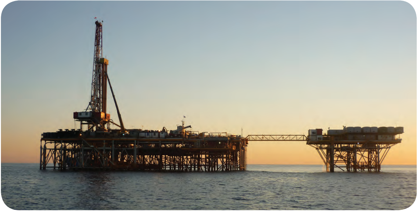
LAM 28 platform, operated by DOTL, located in the Caspian Sea, approx. 25-35km west offshore Cheleken peninsula, Turkmenistan.
