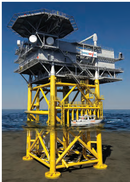
Offshore high voltage substation for Horns Rev C for Energinet.dk currently under construction at HSM Yard, Schiedam, NL.
