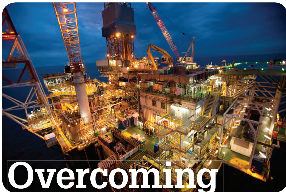
BP's Shah Deniz facility, which started up 2006. Photo from BP.
