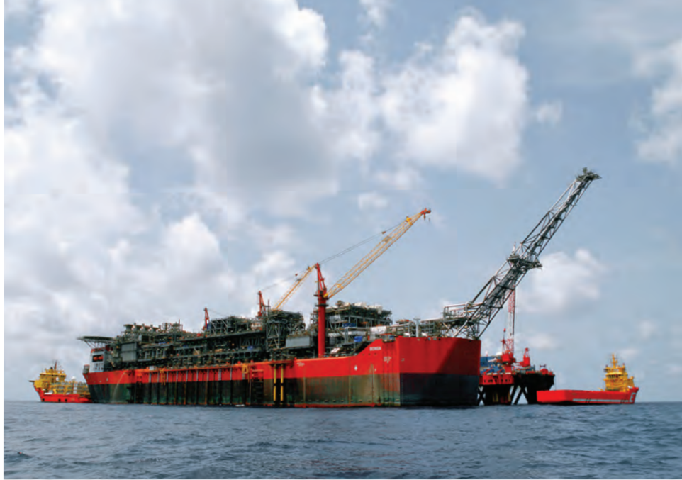
Shell's Bonga North West deepwater project. Photo from Shell.
