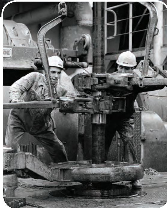
Drilling on Forties in the 1970s. Photo from BP.
