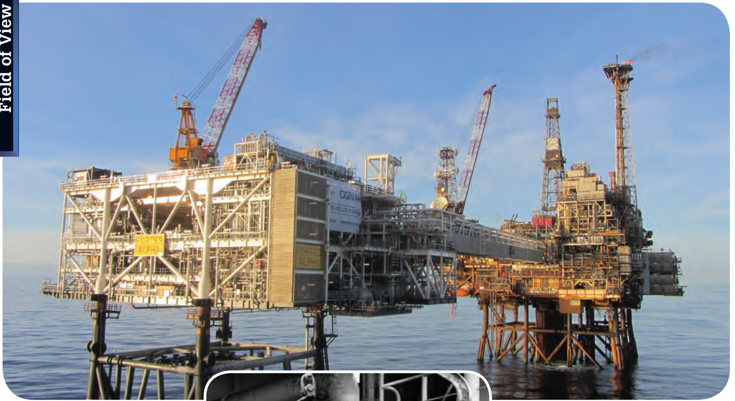
Forties Alpha and the FASP facility. Photo from Apache.
