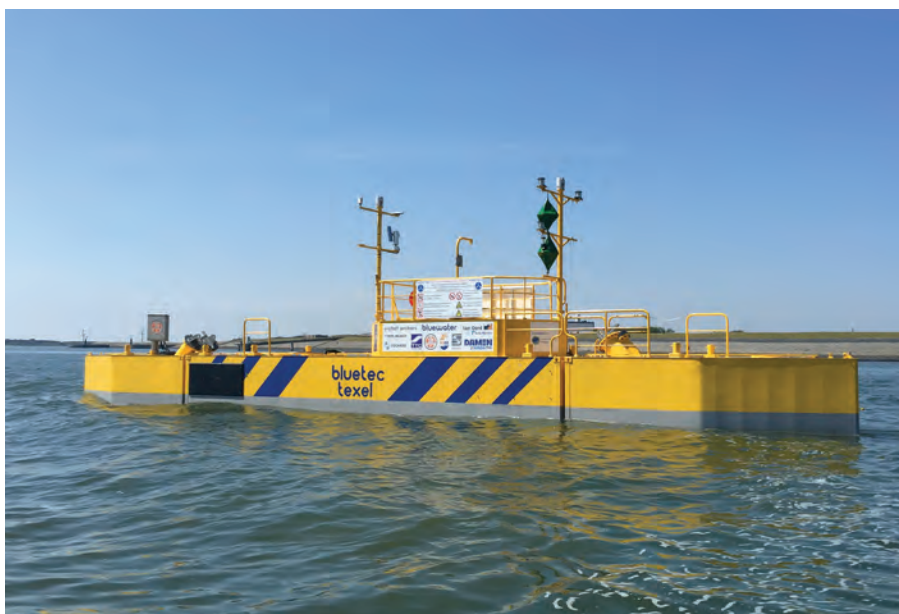
BlueTEC installed offshore Texel. Image from Damen.
