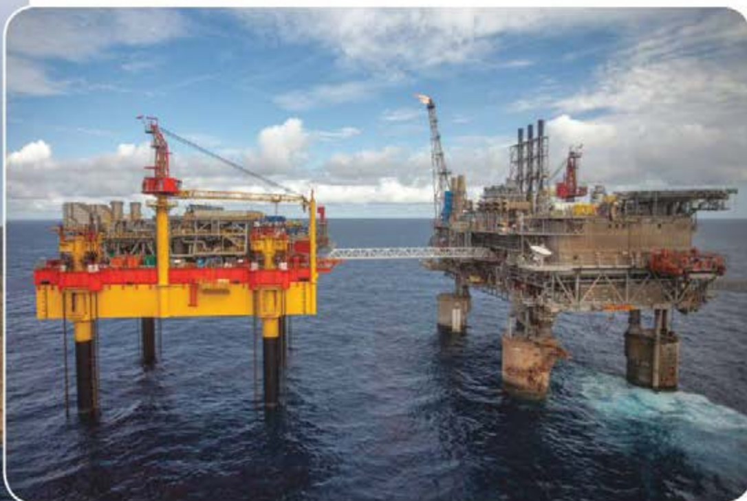
The depletion compression platform was installed alongside the existing Malampaya platform in the West Philippine Sea.
