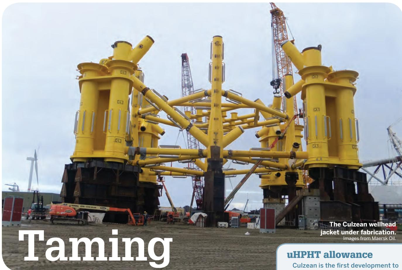
The Culzean wellhead jacket under fabrication. Images from Maersk Oil.
