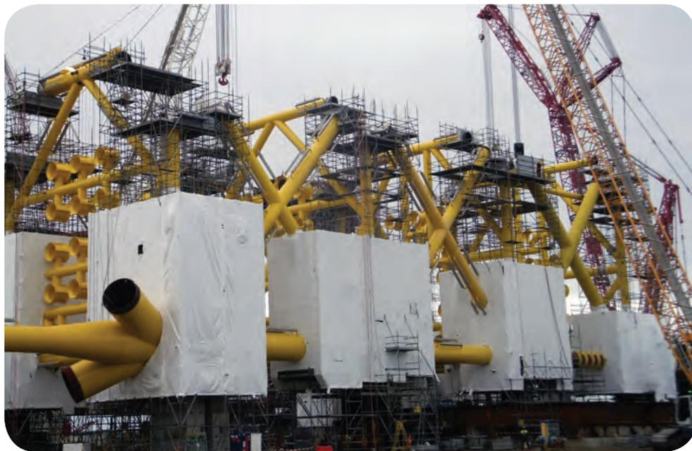
**The Culzean wellhead jacket under fabrication.**
