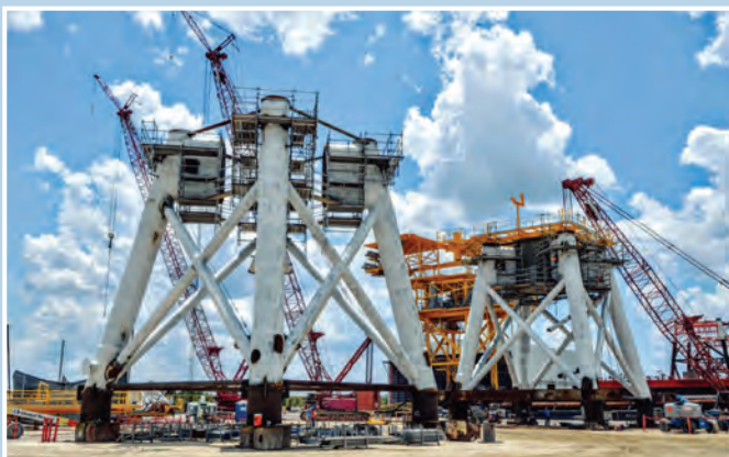
Foundations for Deepwater Wind’s offshore wind farm near Block Island, designed by Keystone Engineering, and built by Gulf Island Fabrication in Houma, Louisiana. This is the US’s first offshore wind farm. Photos from Keystone Engineering.
