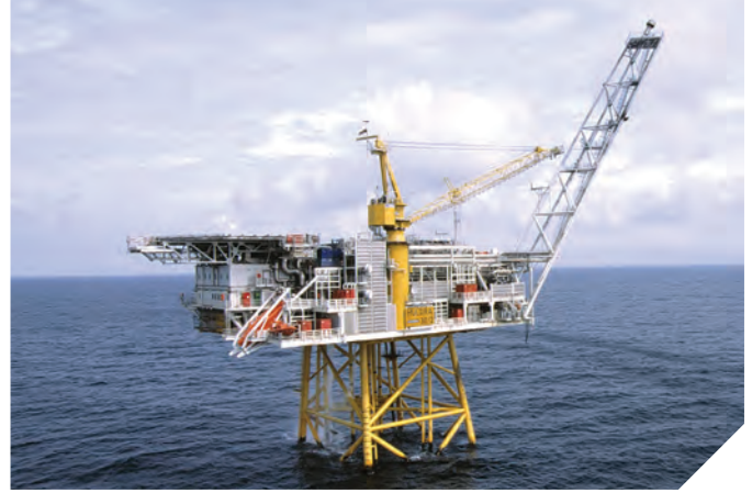
Statoil's Huldra platform, which has been used to help verify DNV GL's P&A guidelines, and resulted in 30-40% well P&A cost savings. Photo from Statoil/Kjetil Alsвик.
