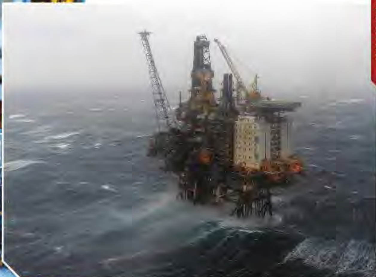
Wintershall's Brage platform.
