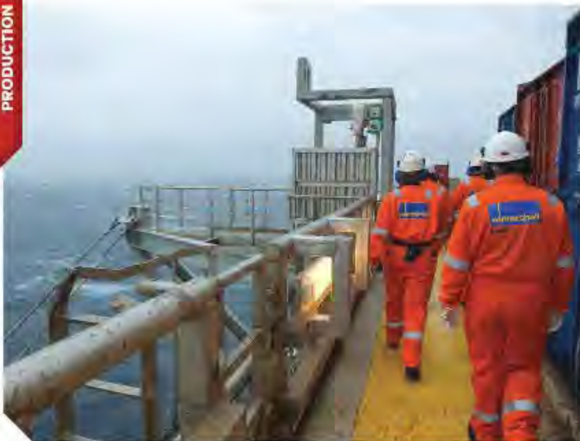
Wintershall's Brage platform.
