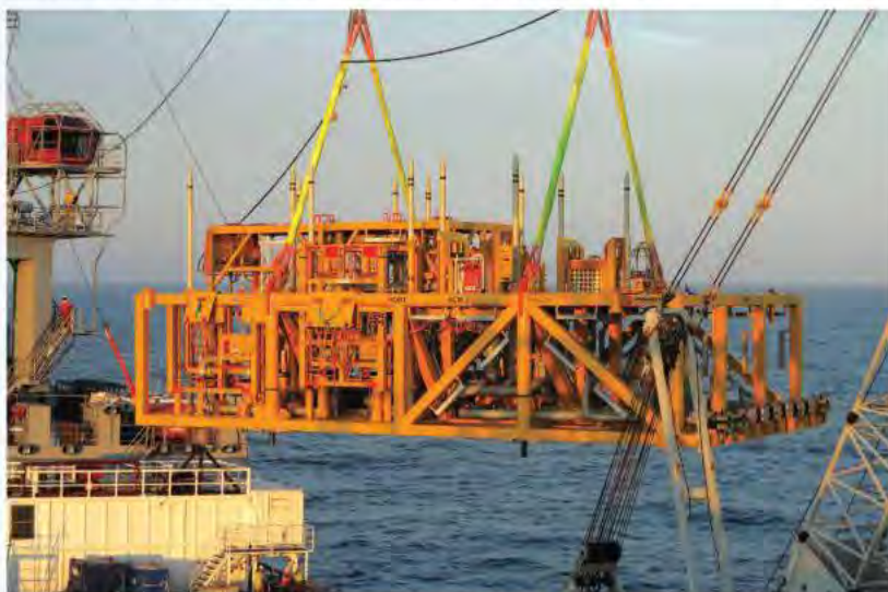
The multiphase compressor station during installation. Photos from OneSubsea.
