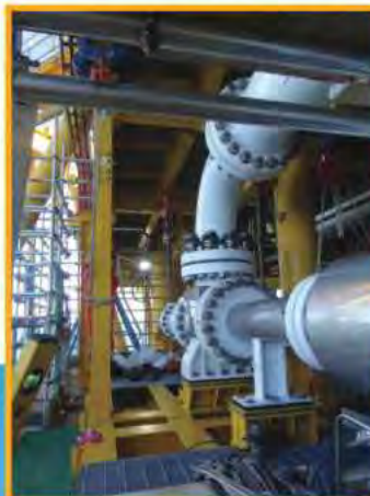
Eductor and Cantilever Sections 4&5.
