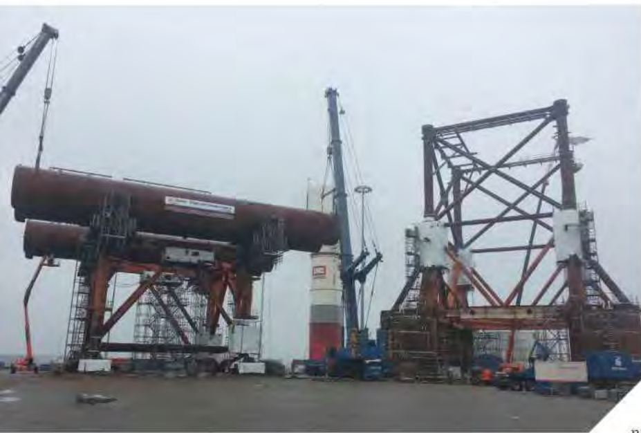
The test platform under construction.
