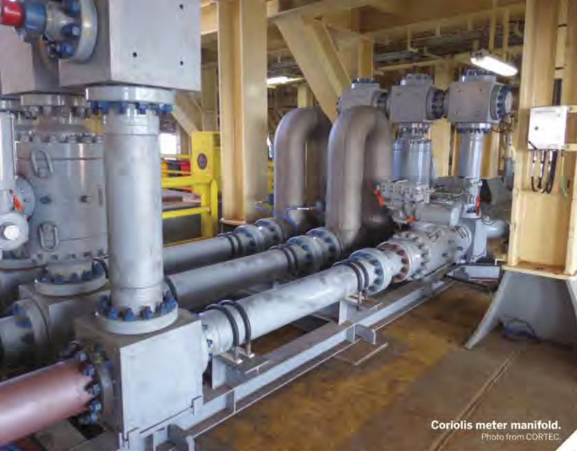
Coriolis meter manifold.
