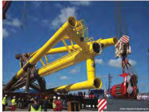
Keystone Engineering's "twisted jacket" foundation to be used on the Atlantic City Wind Farm.
