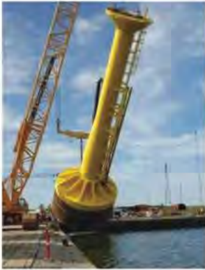
LEEDCo's mono bucket foundation. Photo from DOE.
