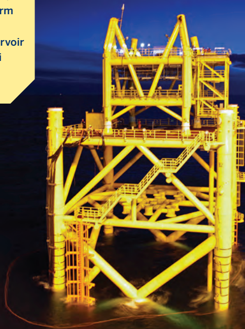
The wellhead platform jacket installed.
