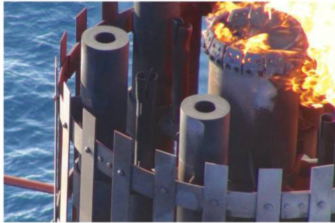
Flare stack inspection. Image from Cyberhawk.
