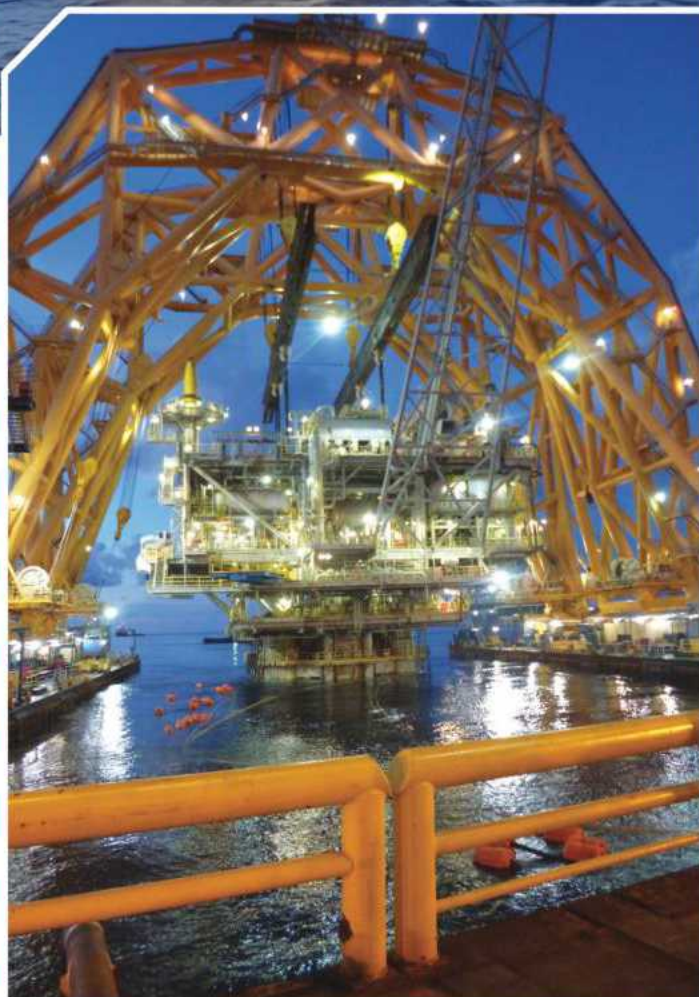
Anadarko's Red Hawk topsides lifted off towing. Photos from InterMoor.
