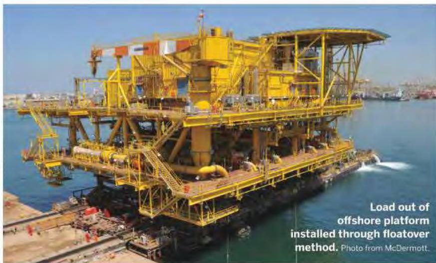
Load out of offshore platform installed through floatover method. Photo from McDermott.
