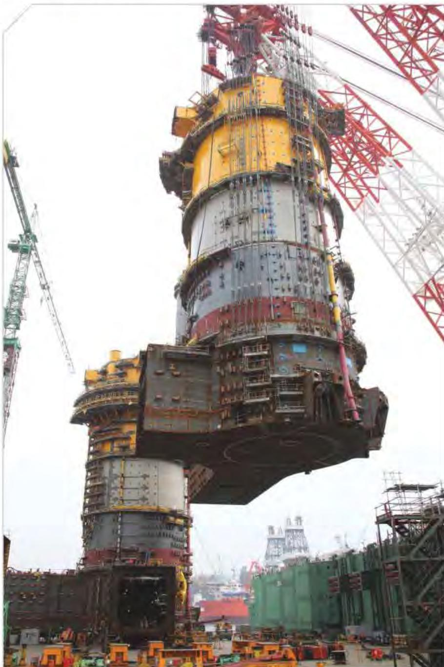
**In February 2016, massive columns known as giga blocks used for the construction of the TLP hull, were lifted into the offshore floating dock at SHI on Geoje Island, Korea. Over an 18-month period, the hull was fabricated, lifted, assembled, and mechanical activities completed.**
