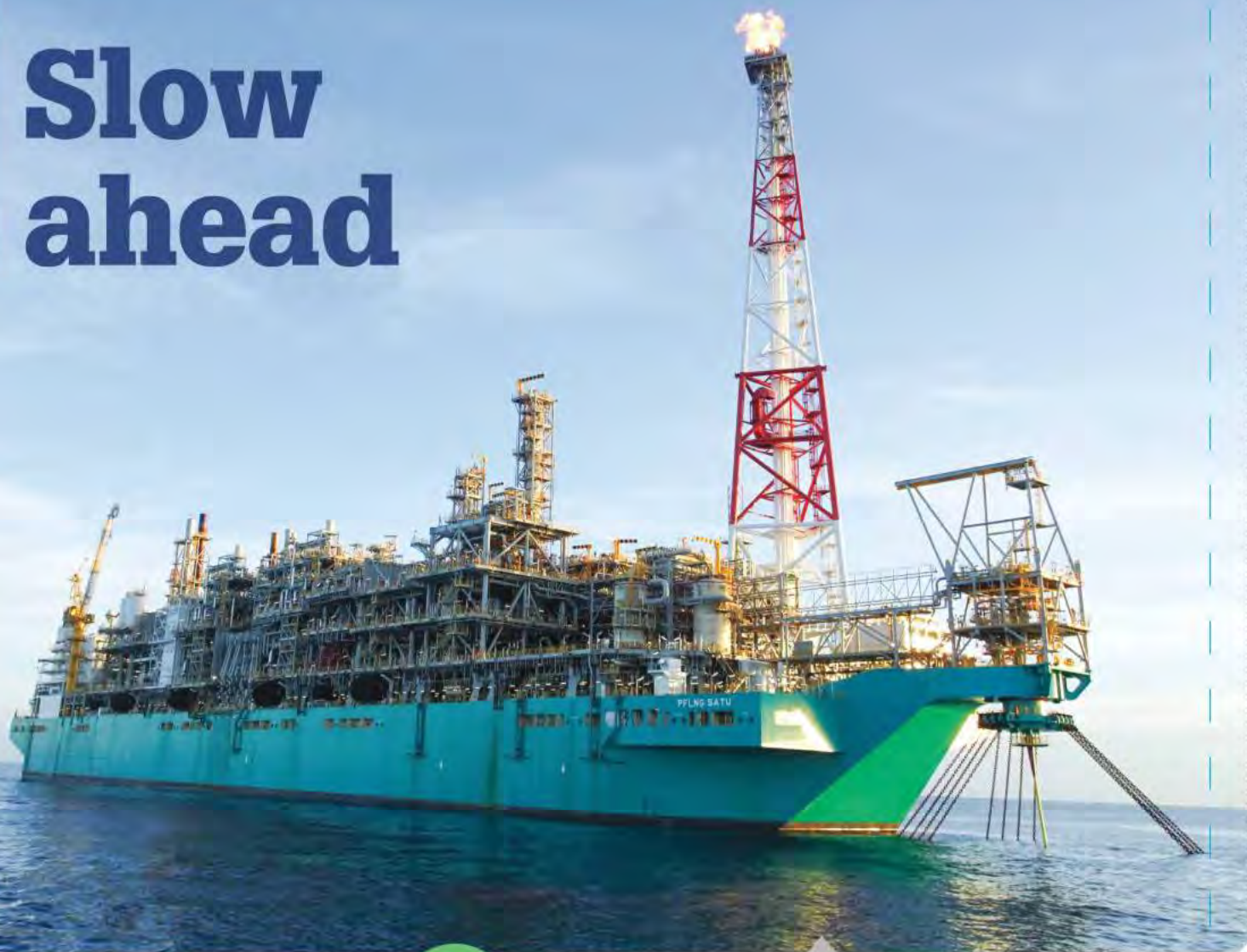
Petronas' PFLNG Satu. Photo from Petronas.
