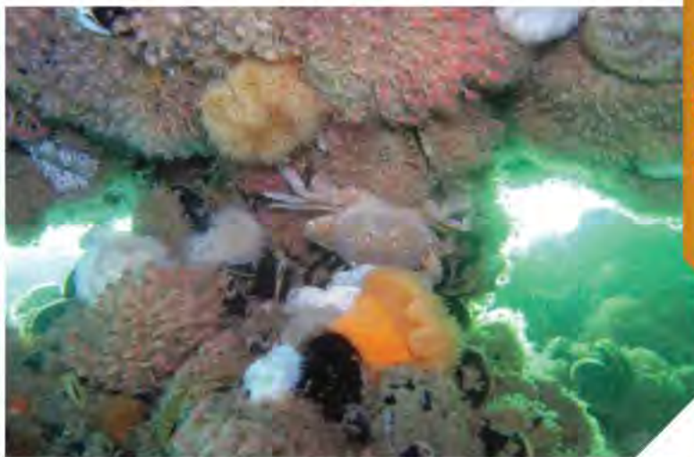
Piles with fouling community that develops on the deeper part of structures, such as anemones, other cnidaria and blue mussels.
