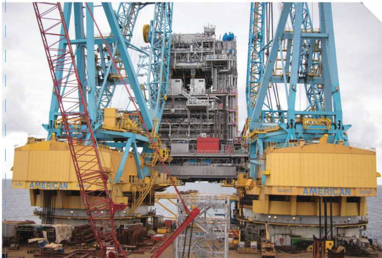
Installation work using the Saipem 7000.
