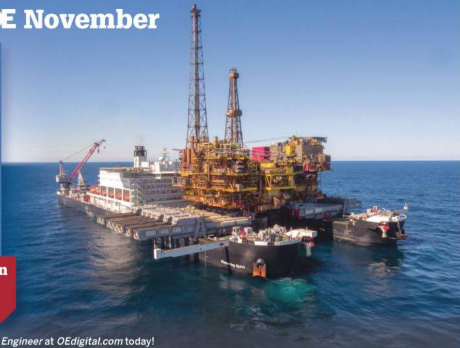
Brent Delta topsides removal. Photo from Shell.
