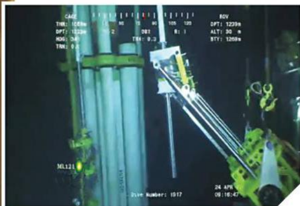
Above: Image from the installation phase. Left: The connector installation frame and anchor gripper unit, onshore assembly. Images from Connector Subsea Solutions.
