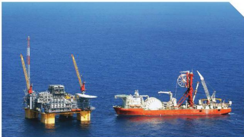
Deep Blue working alongside Shell's Na Kika platform in the Gulf of Mexico.
