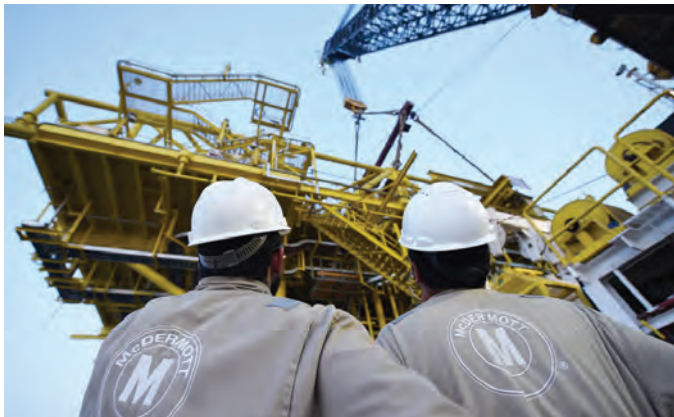
Platform installation in progress. Photos from McDermott.
