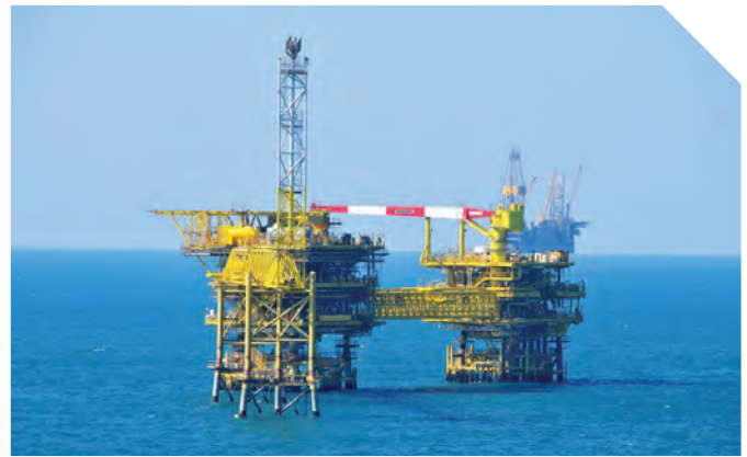
Oil and gas installations offshore Saudi Arabia.
