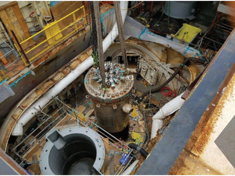
The reactor pressure vessel aboard the STURGIS, the Army's retired floating nuclear power plant recently decommissioned, is carefully lifted in order to be placed in the specially designed shielded shipping container to its left at the end of May 2017.
